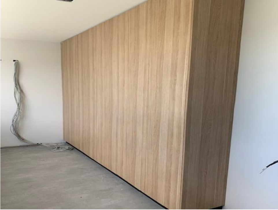
Cabinetry to office
