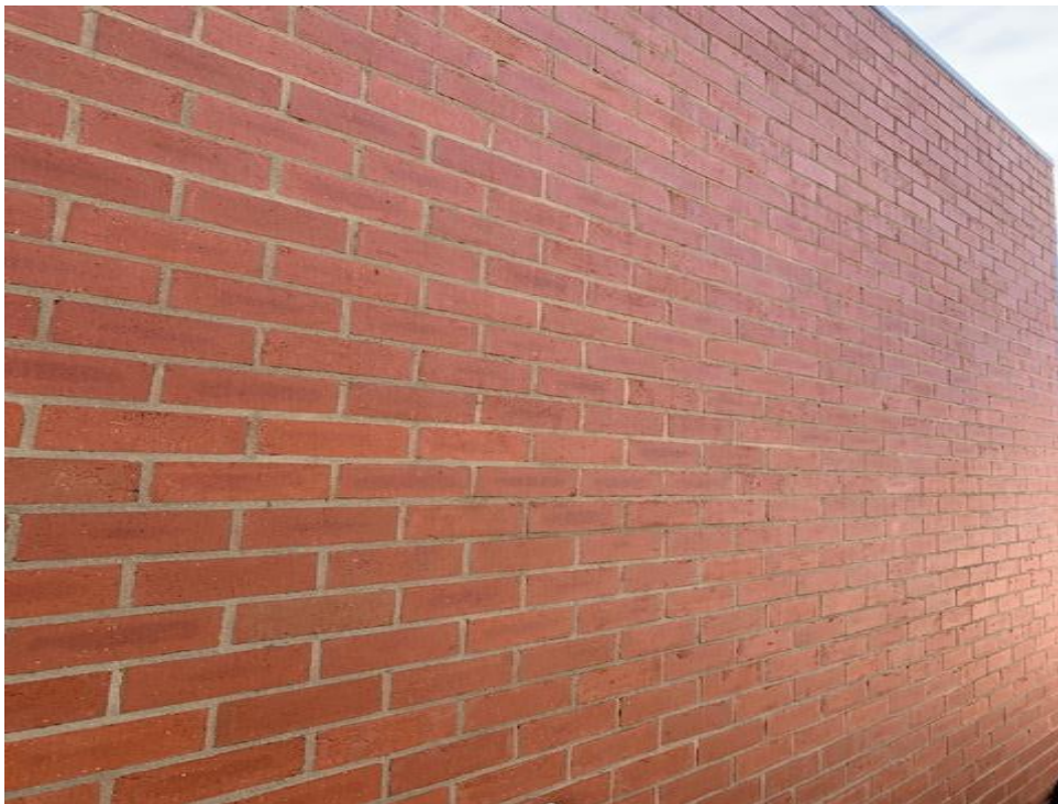
Cleaned Red Bricks
