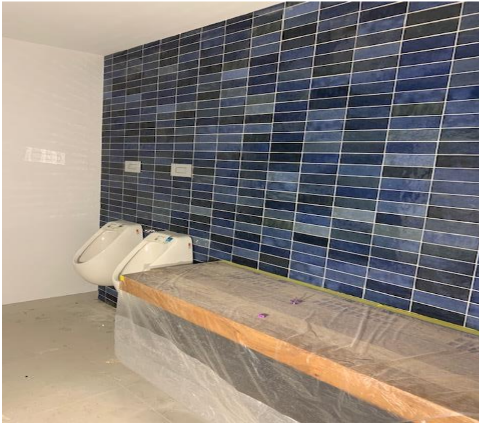
Sneak peak at the Tiling and Joinery to the toilets
