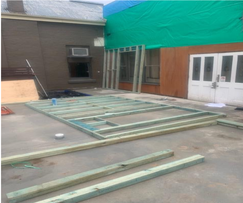
Photo 2: Framing Works Are Underway...!
