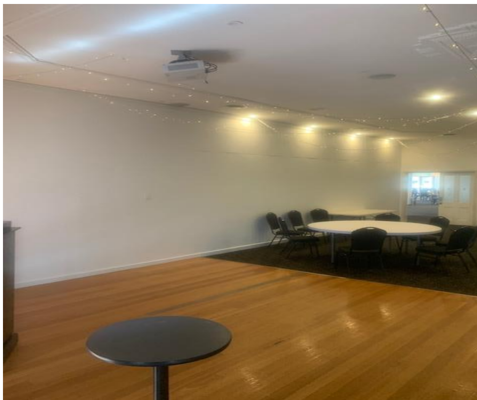
Photo 1: Temporary Wall To Naismith Room
